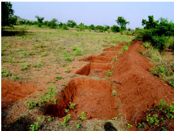
Construction of bund for Chandegutta was undertaken under NREGA in 2006. As a result of the elevated bund, water holding capacity of the bund increased and water accumulated making it available even in summer.
