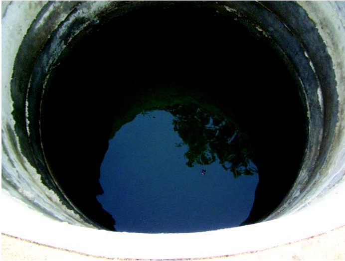
This ring well was constructed with Vikalpa's support in Gurlaguda village of Baddokla GP at a cost of Rs.33,000 and belongs to Teertha Sagaria. This well has a diameter of 8 ft. and a depth of 20 ft. It irrigates about 2 acres of land
