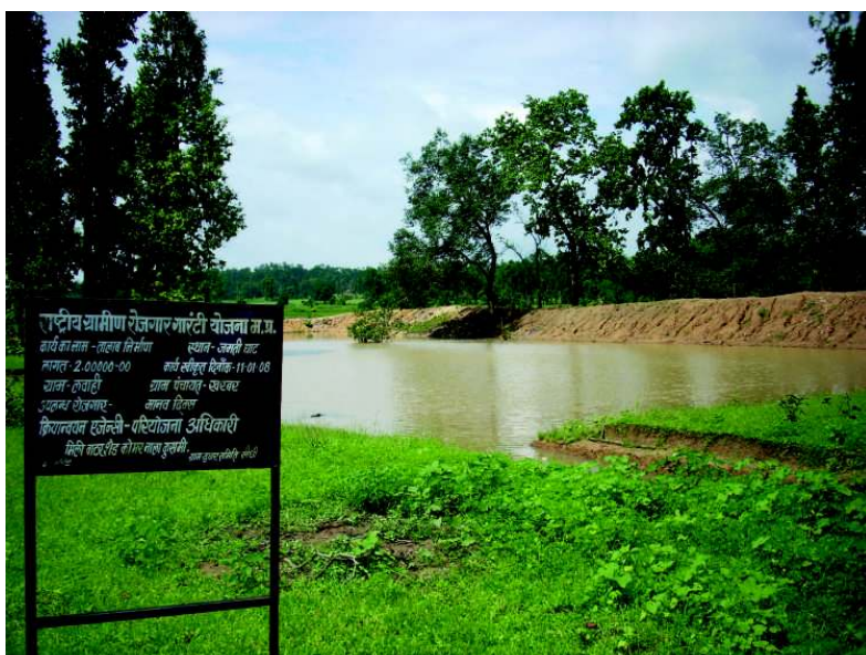
Water fills up after the monsoon in these earthen water harvesting structures built with the support of Gram Sudhar Samiti
